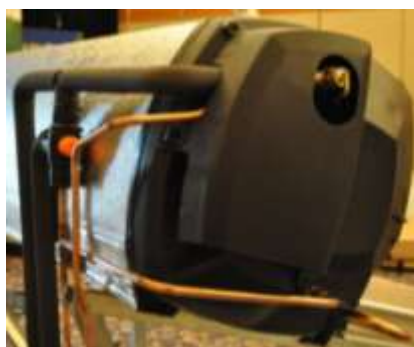
Installation without a HartStat Over Temperature Protection System
