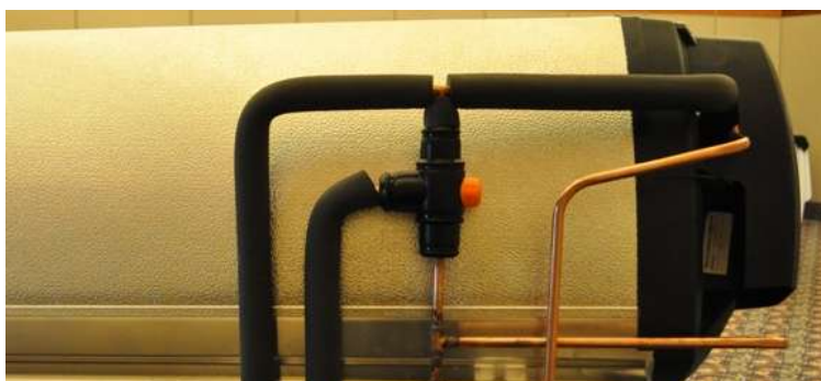
Installation without a HartStat Over Temperature Protection System
